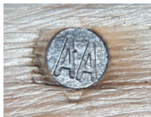
Fig.: 10: Nail picture "certified nails"
